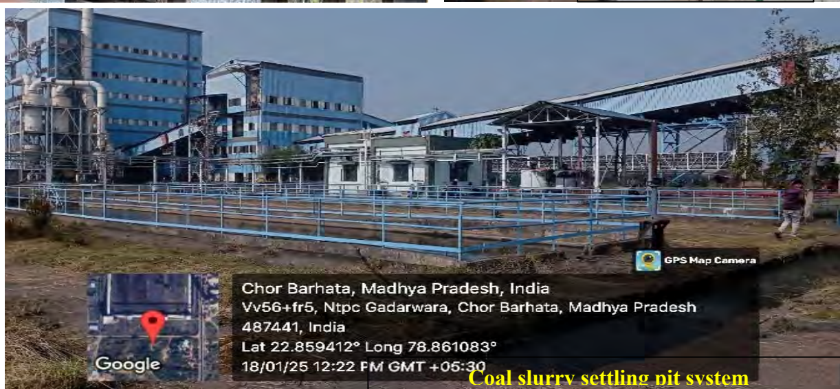
Figure 6.1 Infrastructure at Plant
