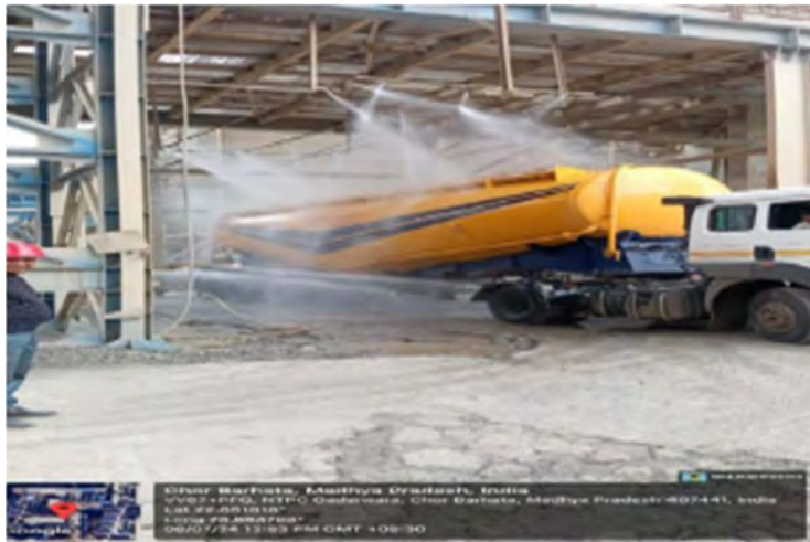
Water Sprinklers at Ash Silo
