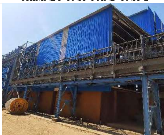
GYPSUM SHED (GYPSUM HANDLING SYSTEM FOR BOTH UNITS)
