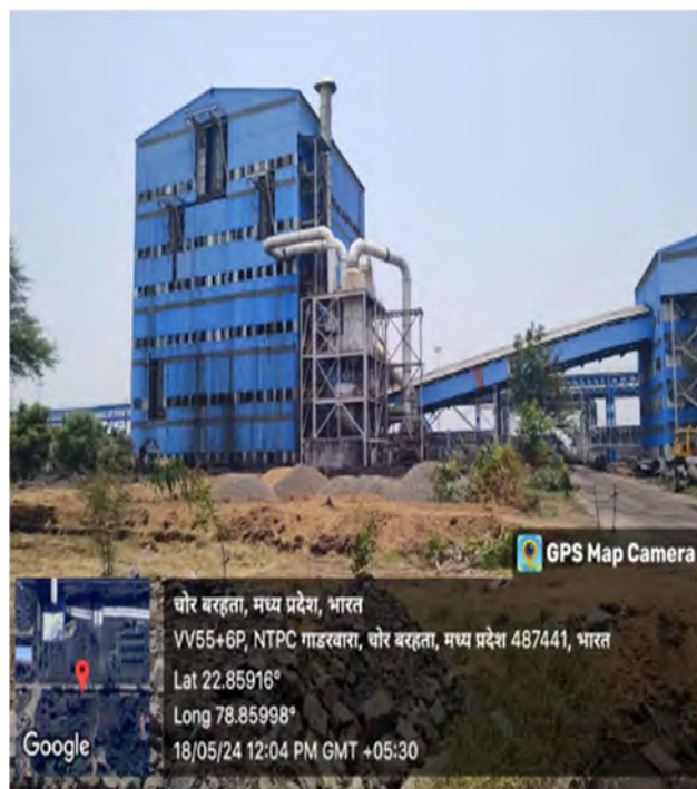
Dust Extraction & Suppression at Coal Crusher House
