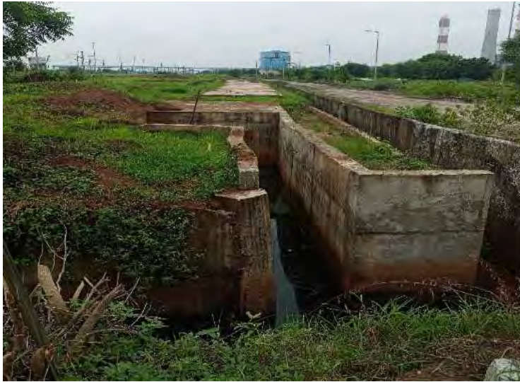
Storm water diversion
