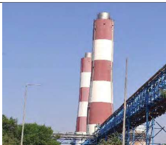
CHIMNEY UNIT-1 AND UNIT-2
