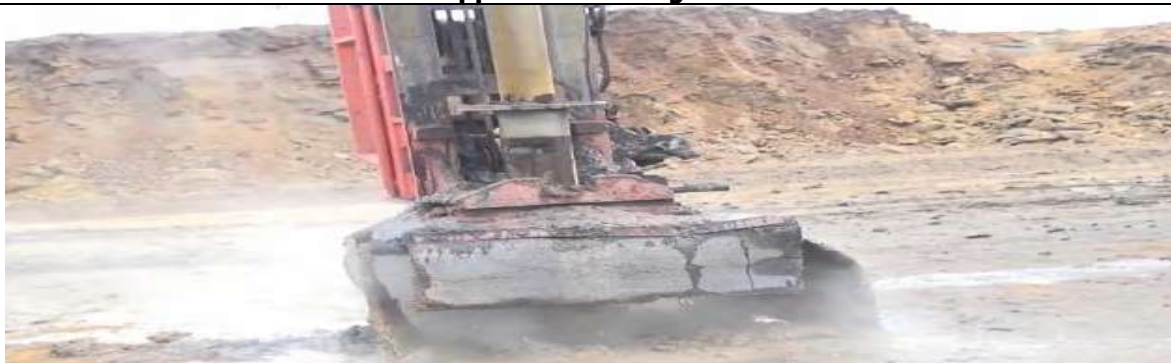
Wet Drilling Arrangement
