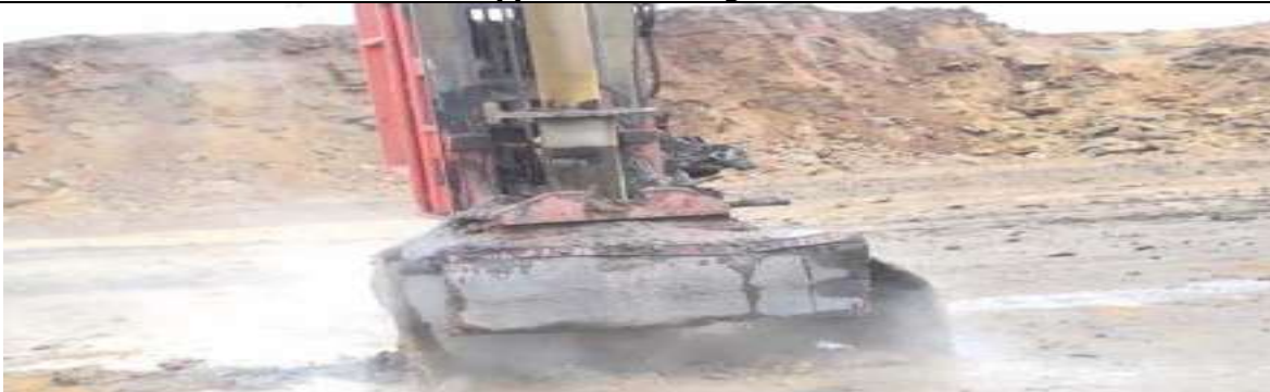
Wet Drilling Arrangement
