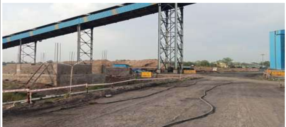
Dust suppression on haul roads near CHP
