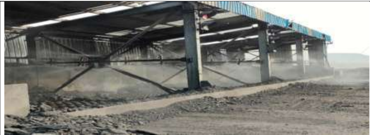
Dust Suppression at Receiving Hopper
