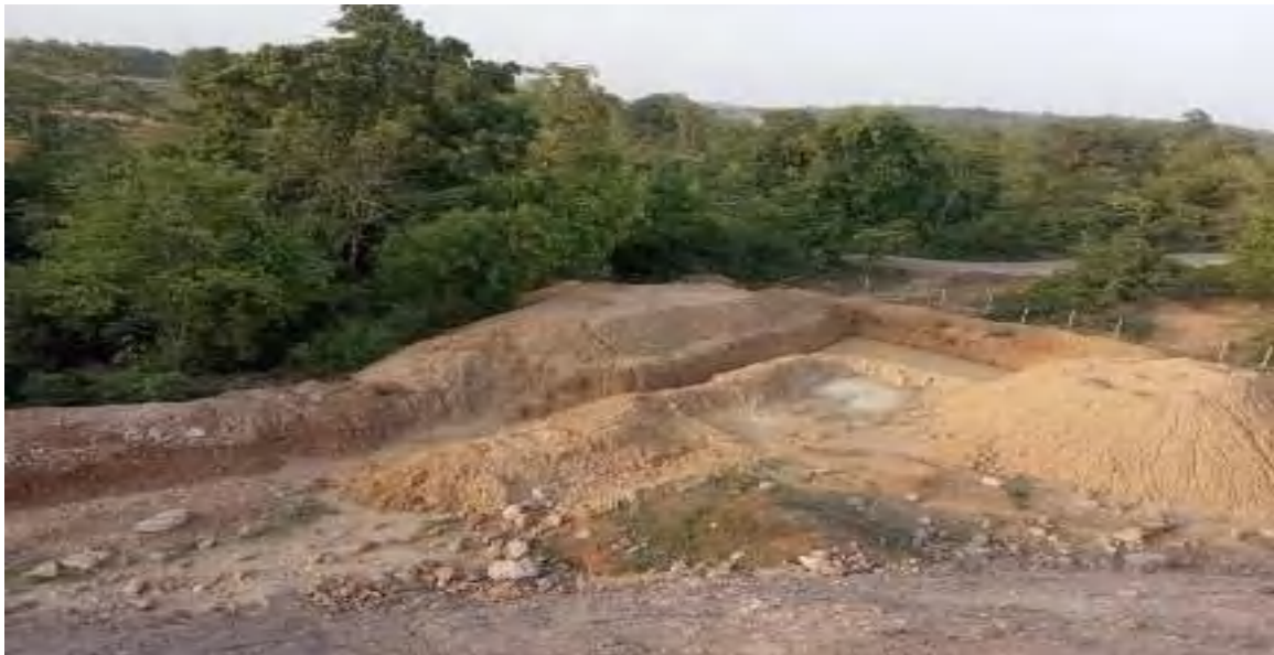
Garland Drain connected to settling pond
