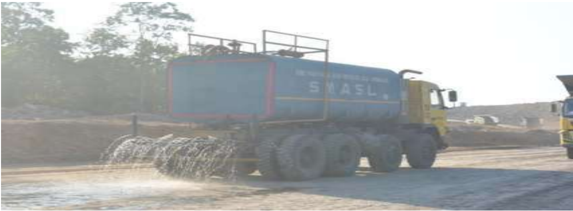
Water Sprinkling on Haul Roads inside Mines
