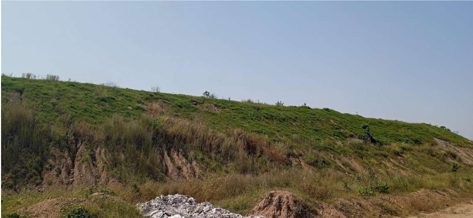
After Grassing Activities along slope of Top Soil.
