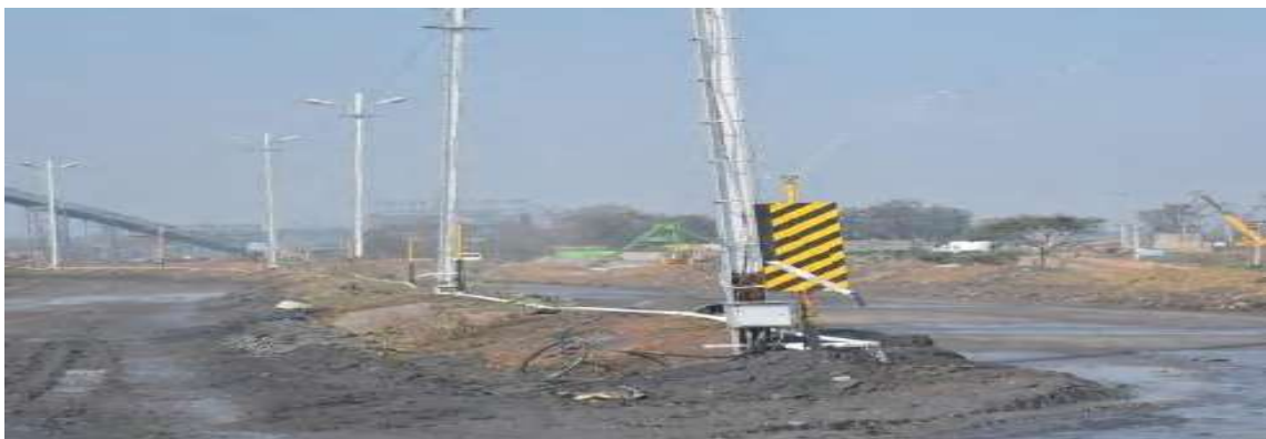
Fixed Type Sprinkling on Haul Roads Near CHP
