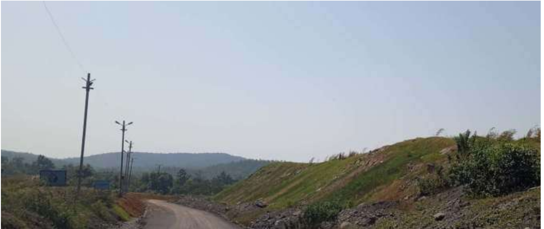
Grassing Activities along slope of Non-Active Overburden Dump.
