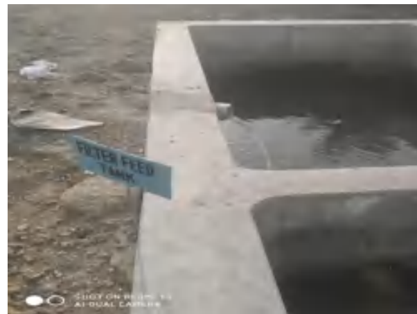
Filter Feed Tank
