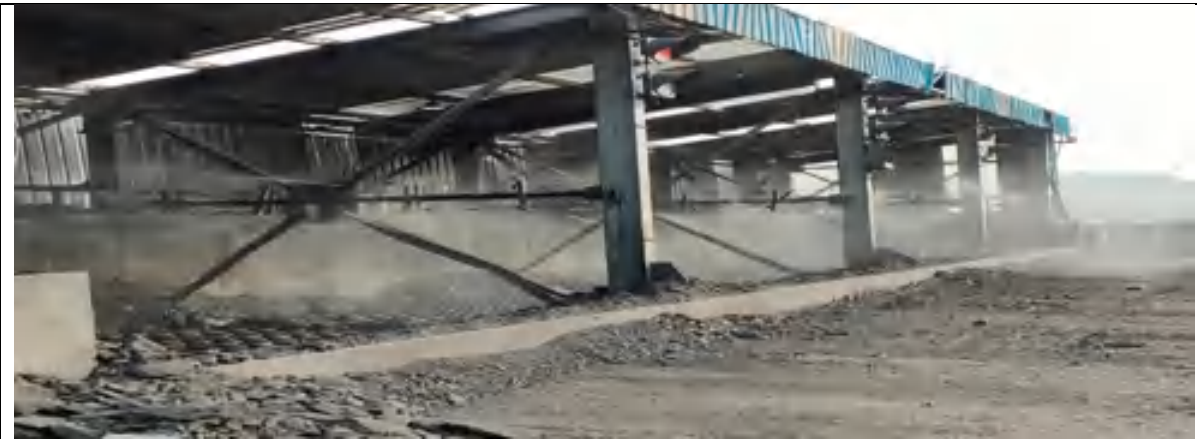
Dust Suppression at Receiving Hopper
