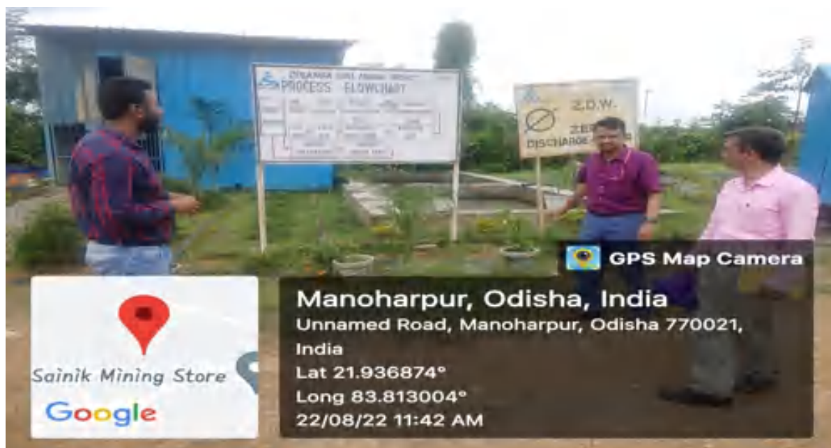
Sewerage Treatment Plant
