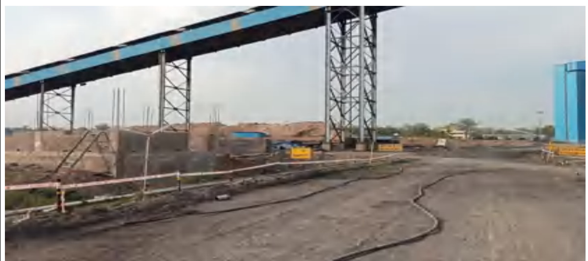
Dust suppression on haul roads near CHP
